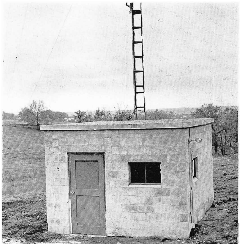
FIG. 13. Transmitter building showing center tower in rear. Note compactness of building and inexpensive type of construction which is typical for remote operation.
