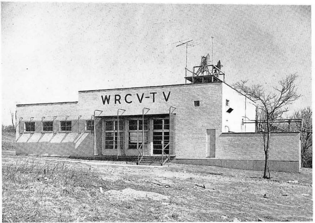
FIG. 11. WRCV-TV has constructed this new transmitter building that incorporates many desirable features, including a garage, a complete workshop, a complete kitchen, and ample office area.
