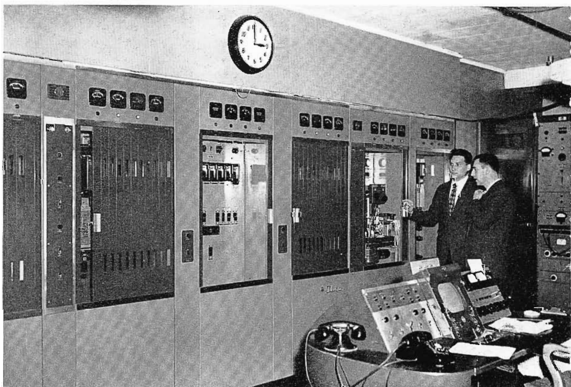
FIG. 8. The 12-kilowatt transmitter installation. The false wall has been removed to provide space for the extra cabinets.
