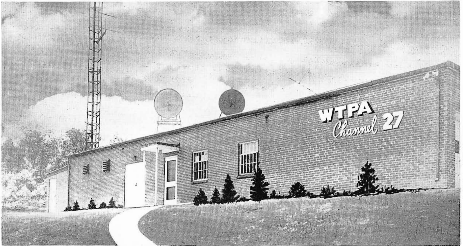
FIG. 5. WTPA transmitter building. A standby tower and antenna were used during conversion.
