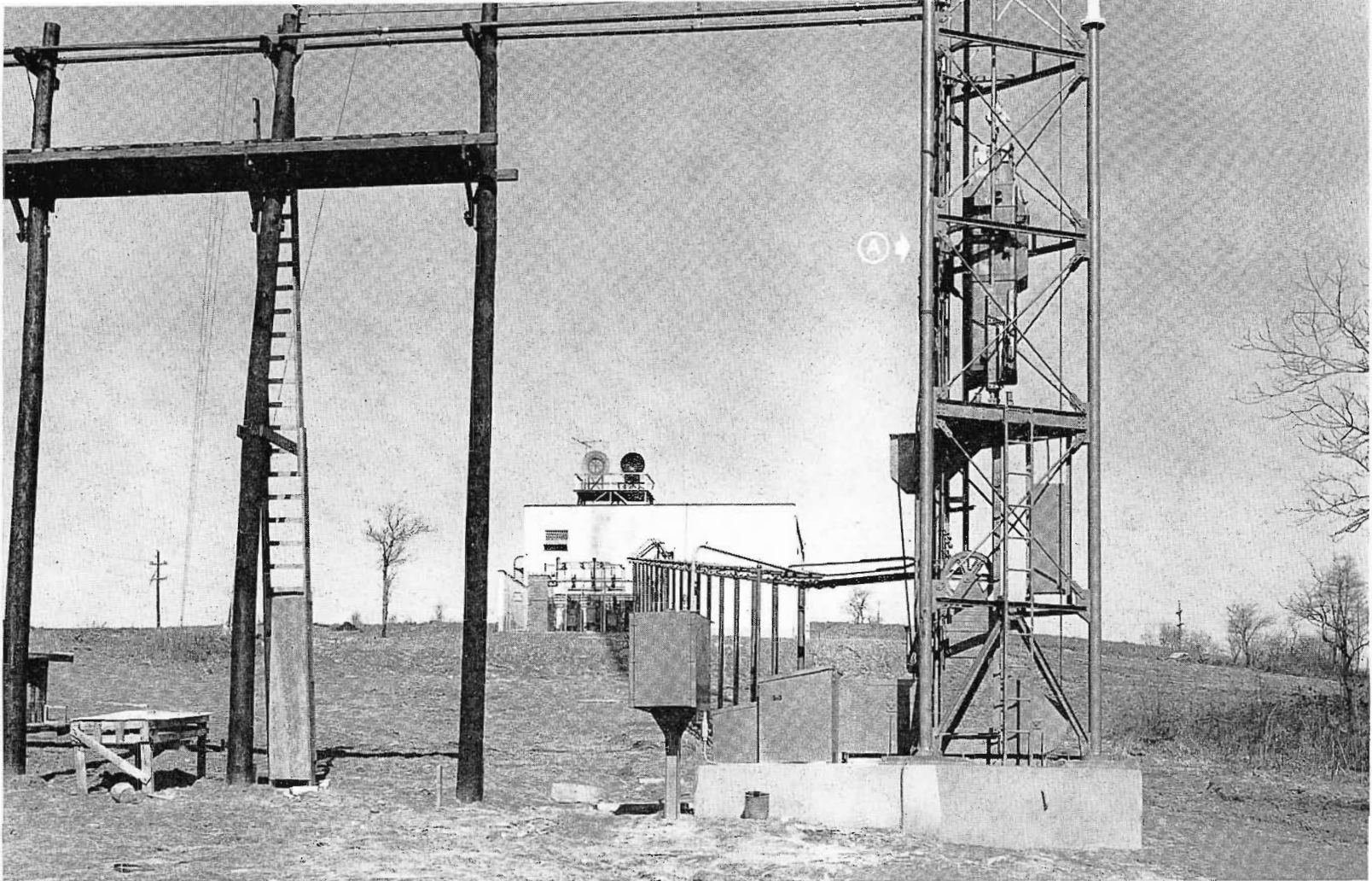
FIG. 4. Base of tower is an 11-foot deep, reinforced concrete foundation, six feet square with only two feet extending above ground. The two-man, radio-controlled elevator, noted by letter A, is shown in above photo.
